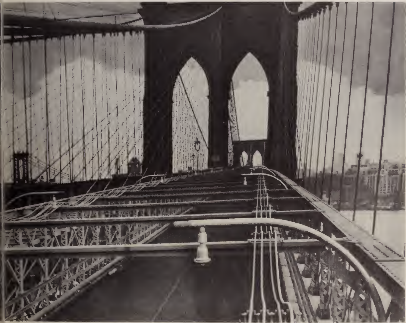
New lighting fixtures and cables were installed on the roadways but the old-fashioned lamps were retained on the pedestrian walk.
